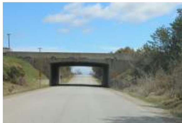
Photo 3: View of the bridge looking west
