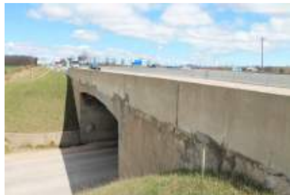
Photo 2: View of the bridge from Highway 400
