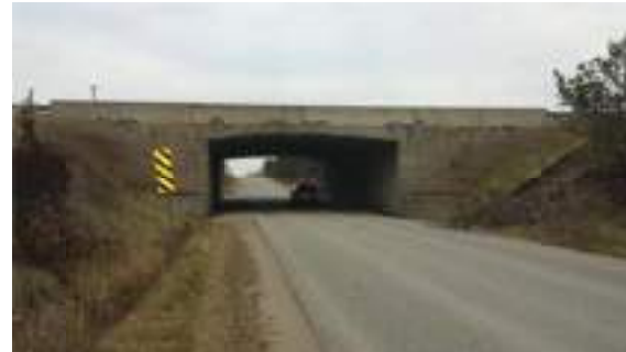
Photo 2: Current Overpass Structure
