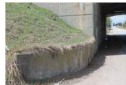
Detail of 6th Line Bridge
