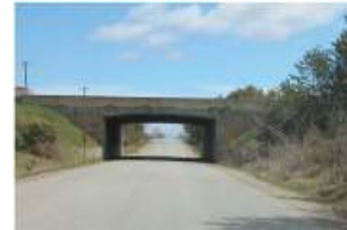
6th Line Bridge as viewed from west
