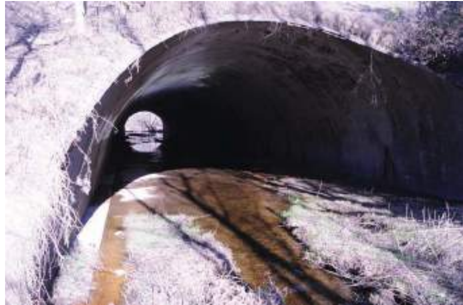
Photo 3: Concrete culvert, view eastward
