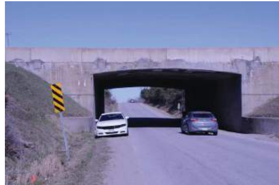
Photo 1: Highway 400 overpass, view eastward
