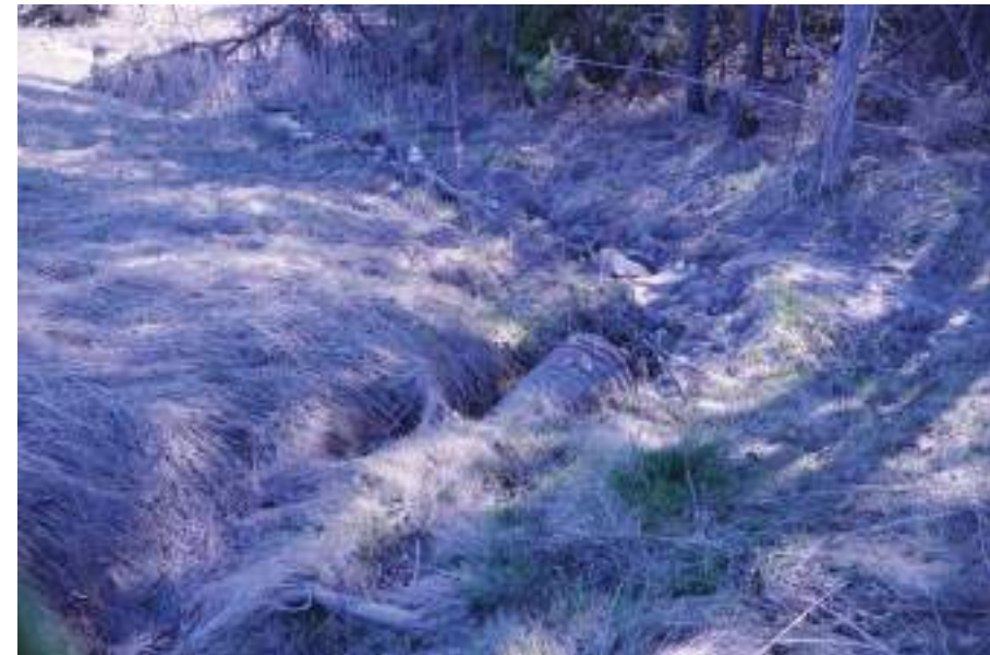
Photo 2: Corrugated steel pipe culvert
