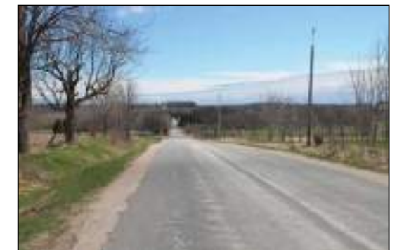
6 th Line looking east from the bridge structure
