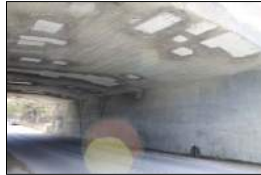
Underside of 6 th Line Bridge
