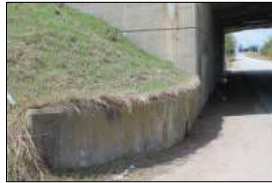
Detail of 6 th Line Bridge abutment
