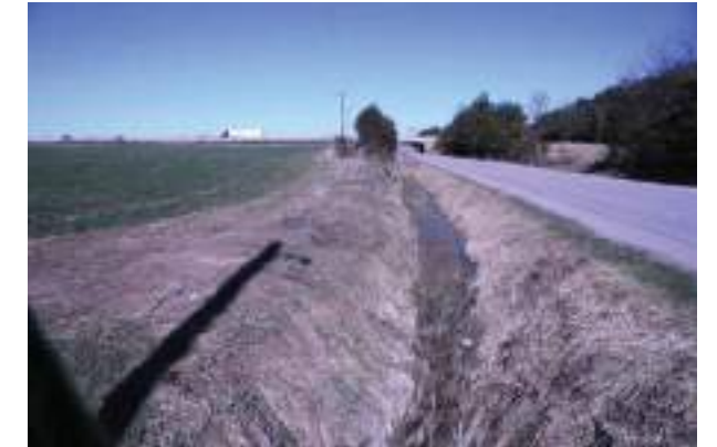
North ditch of 6 th Line west of Highway 400 (in distance) conveying runoff from MTO culvert C-56 just north of the intersection
